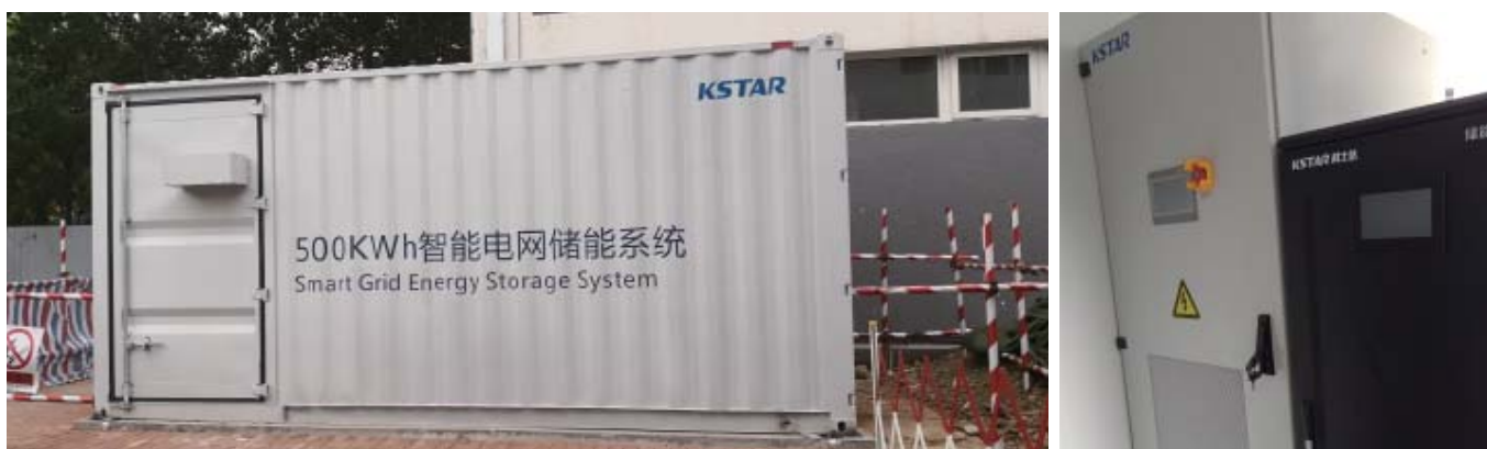
▶▶▶ 500kWh Multi-energy Complementary Project of Beike Industrial Park
