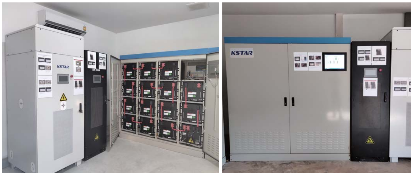
▶▶▶ 100kW/300kWh Micro-grid system in Pong Phang, Thailand
