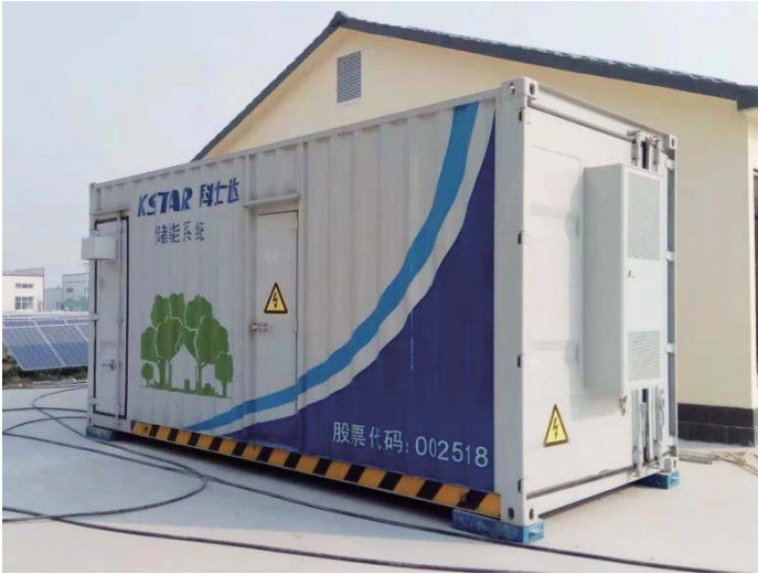
► 50kW/200kWh BESS for EV Charger Station in Hebei
