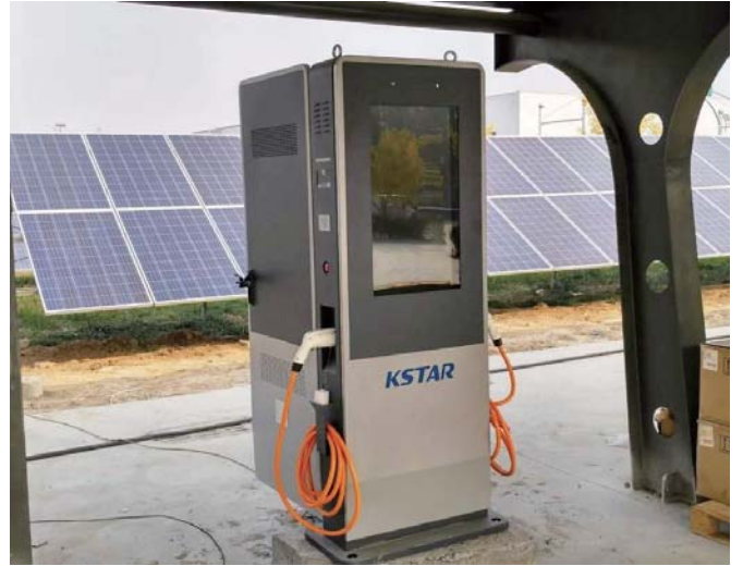
► 50kW/200kWh BESS for EV Charger Station in Hebei
