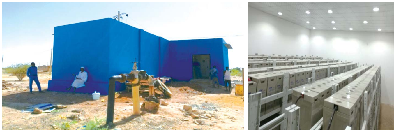
▶▶▶ 300kW/2.16MWh BESS of Off-grid in Sudan
