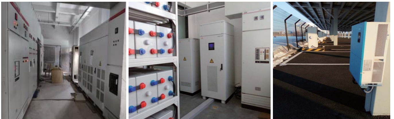
▶▶▶ BESS for EV Charger Station in Harbin
